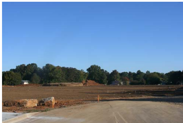
Work progresses 10/7/08 (photo courtesy of 2008 HUGHESHUE.COM)
