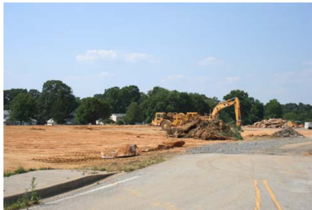
Work has started on the new fields 7/12/08 (photo courtesy of 2008 HUGHESHUE.COM)
